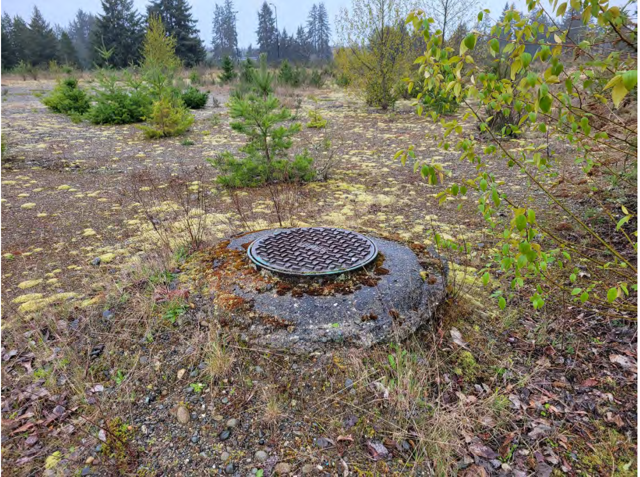
Looking south at a sewer manhole on Lot 3
