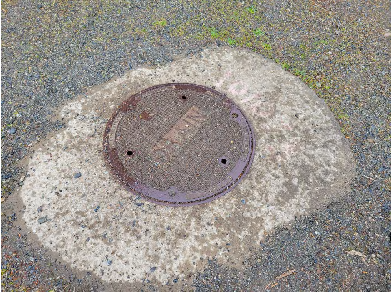
An example of a drain access cap on Lot 5
