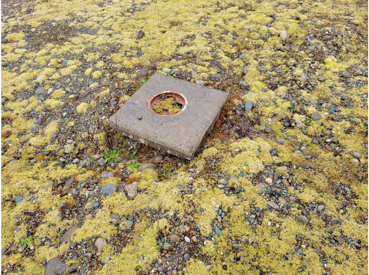
Unidentified concrete and metal cap on Lot 9
